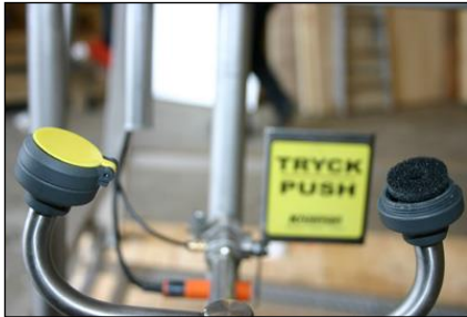
Figure 8: Eyewash spray heads
